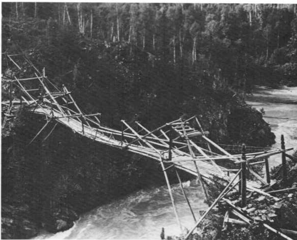
19. Indian suspension bridge used on the Upper Skeena River at Ragwilget village. National Museums of Canada photo 60313.
