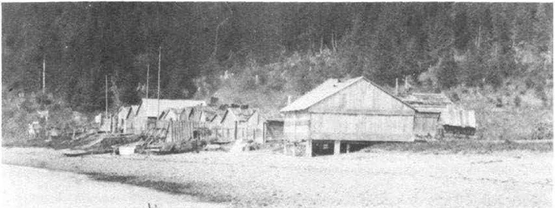
Figure 13 The partially fortified Tlingit village of Hoonah in Southeast Alaska. Only five of fourteen houses have been included within the palisade. The props are only found on the front of the fort and may have been to roll logs down on invaders like at the Kitwanga Ta'awdzep. The house in the foreground is built out beyond the winter high tide line on props like two of the Ta'awdzep houses. On the extreme right behind the village is a brush structure that is probably a sweat lodge. Northwest Trading Company Photo circa 1805. Courtesy Berlin Museum für Völkerkunde. (NMC neg. 78-6040).
