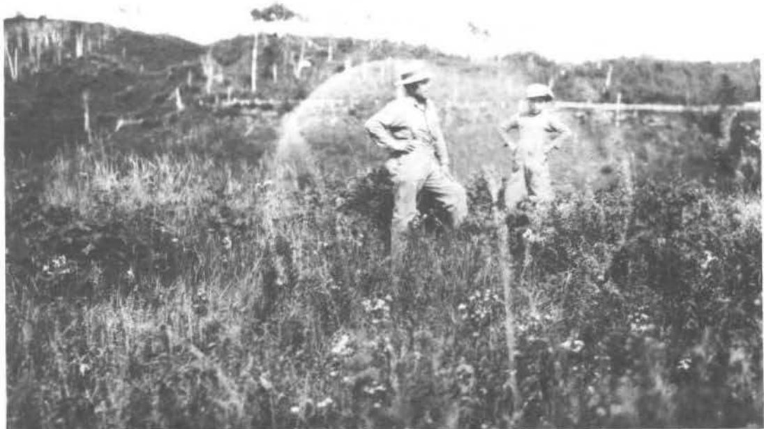
Figure 70 Two Kitwanga people standing in the central pit of Nekt's house, which is the most likely place for the double-floored structure mentioned in the legends. It was the first building on top of Ta'awdzep and was designed to protect the Kitwanga people from Haida invaders. (Photo by Marius Barbeau 1924. NMC 59723).
