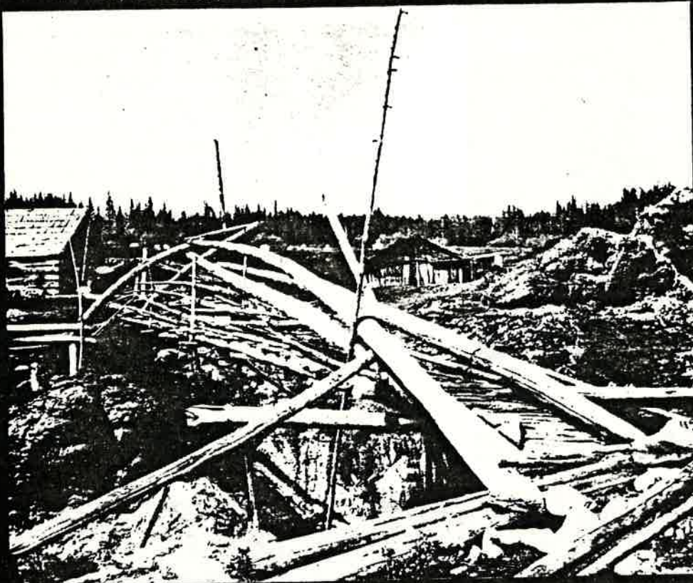
THE SUSPENSION BRIDGE ACROSS THE CANYON, 1899
