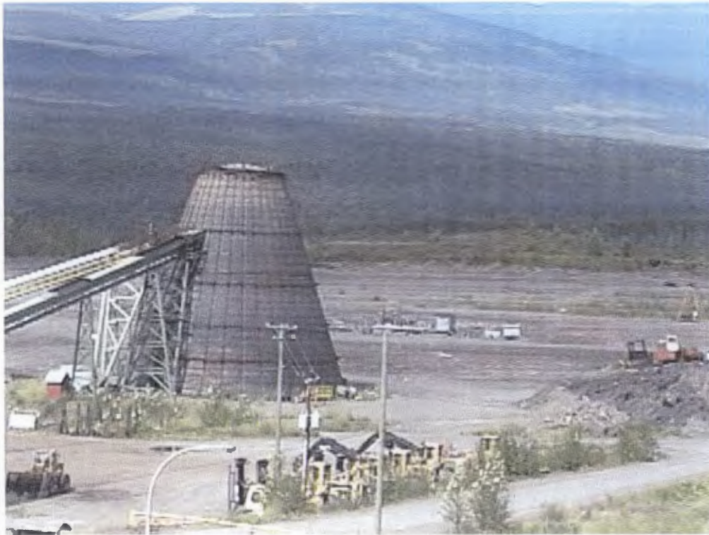
Figure 4: The Mill at Carnaby no Longer in Operation.
